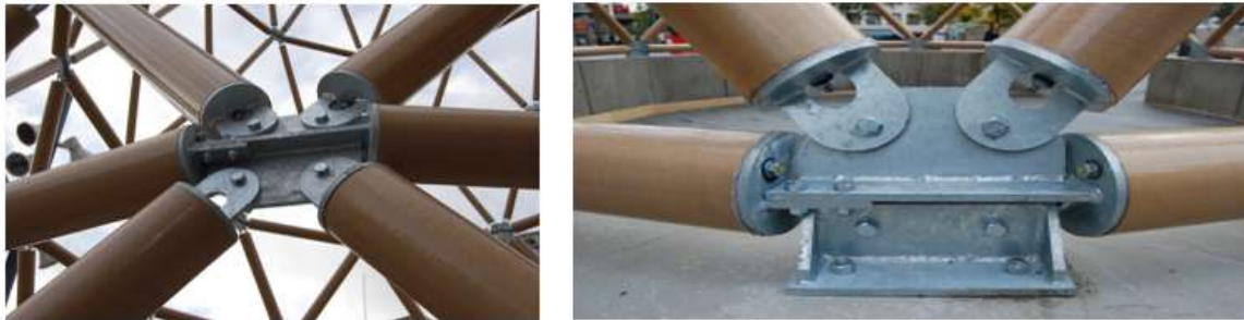
Figura 17. Uniones en acero utilizadas en la torre de cartón tubular en el London Design Festival 2009 Tomado de: WordPress.com. (s.f.). SHIGERU BAN: BUILDING WITH PAPER – BOATHOUSE AND PAPER TOWER. Recuperado de https://clarewashington.wordpress.com/2012/12/10/shigeru-ban-building-with-paper-boathouse-and-paper-tower/ .
