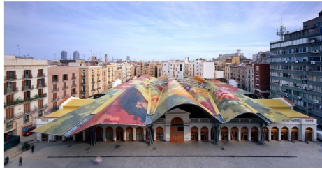
Figura 55: Fachada principal plaza Santa Caterine
