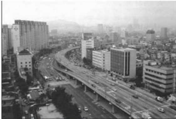
Autopista Cheonggye Expressway (1999)
