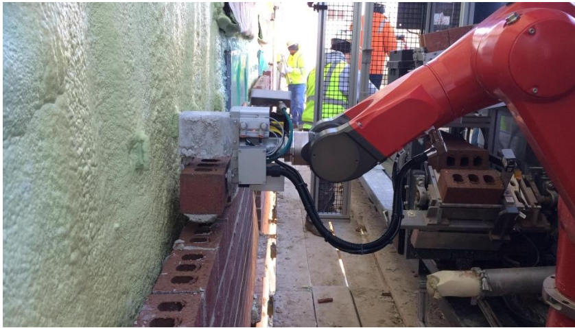
Figura 2: SAM 100. 2007. El robot albañil. Tomado de “Construction Robotics” por Construction Robotics Advancing Construction, 2007, recuperado de https://www.construction-robotics.com/sam100/
